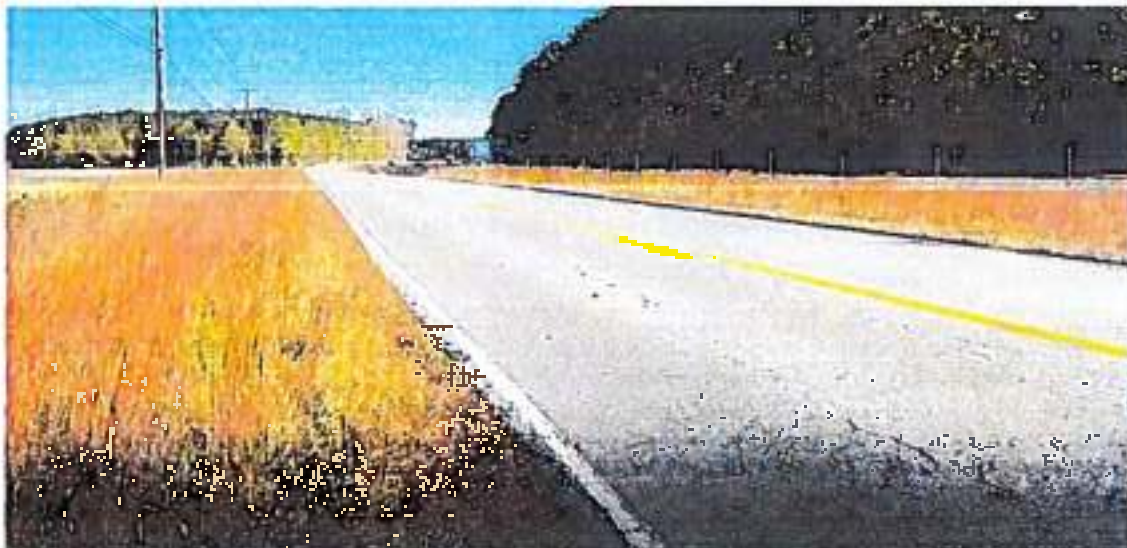
Figure 4 – Blue Star Highway adjacent to subject parcel
