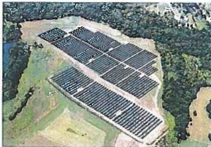
Figure 1: Utility-scale solar facility (AP100) located in Cherokee County. Source: StreetView
