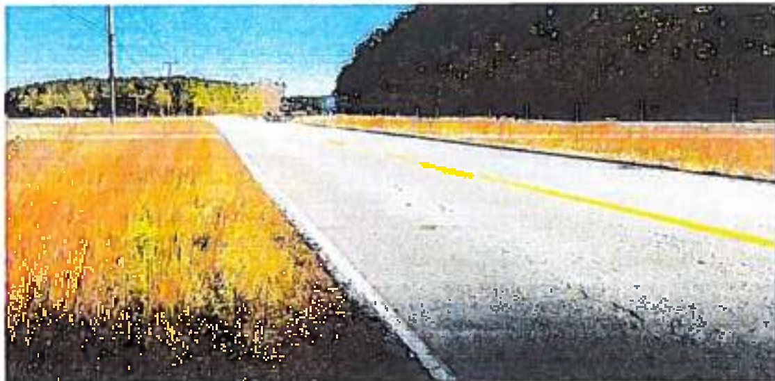
Figure 4 – Blue Star Highway adjacent to subject parcel
