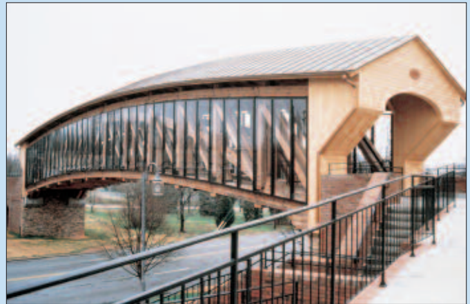
Old Salem Covered Bridge; Winston-Salem, North Carolina (courtesy of Blue Ridge Timberwrights)
