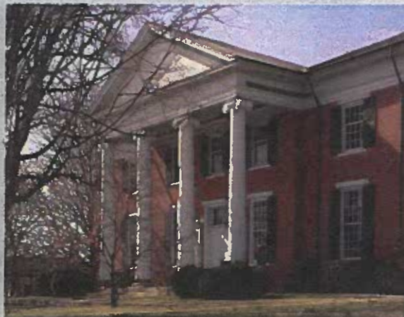
Halifax County Courthouse, 1839.
