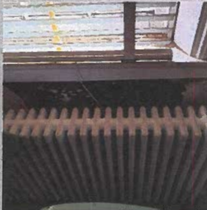
Section of wall plaster missing from wall.
