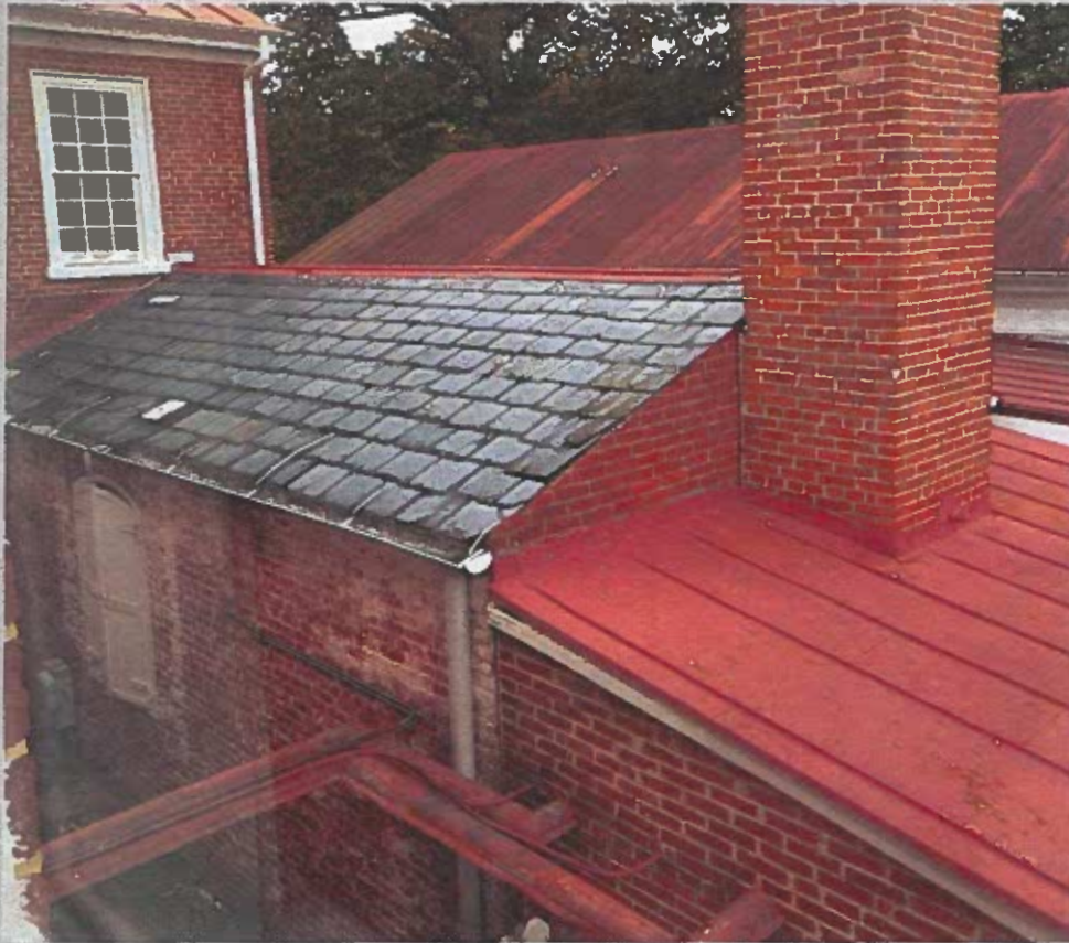
1893 Clerk's Office Vault in its present-day condition.
