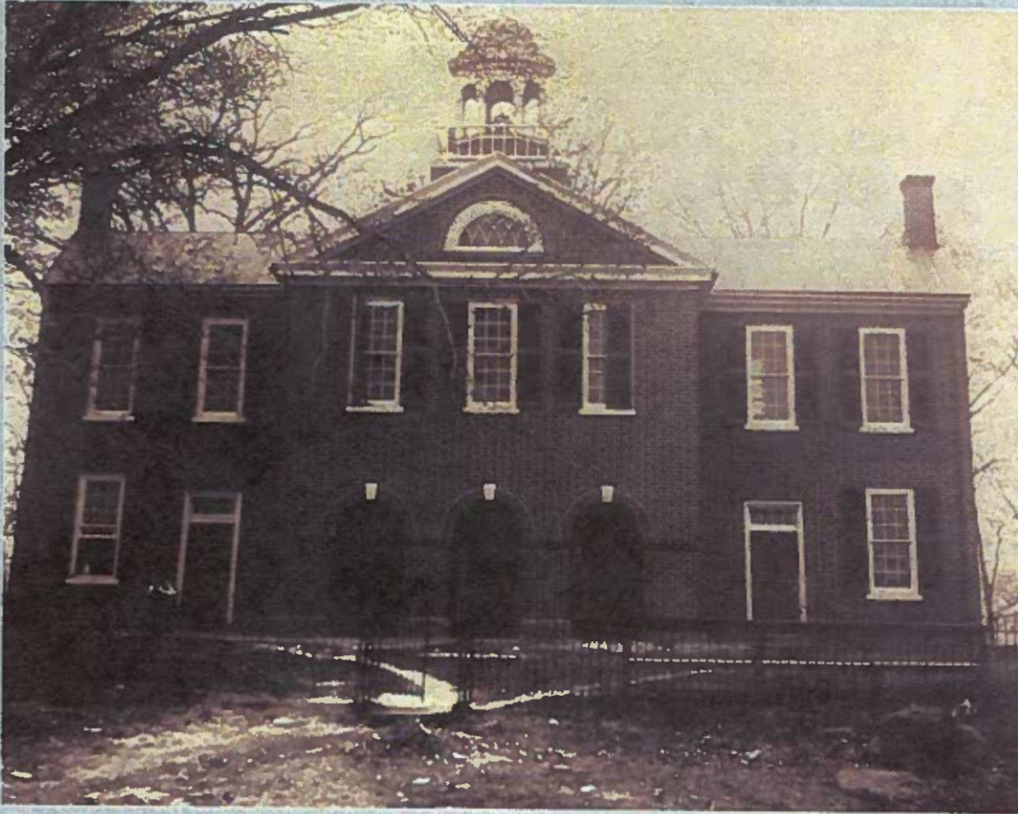
Sussex County Courthouse after 1912, shows the brick to be in good conditions, other than a stuccoed base where there may have been moisture damage to conceal.
