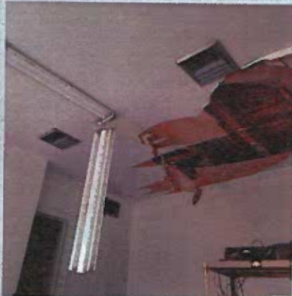
Existing ceiling condition in 1954 addition.
