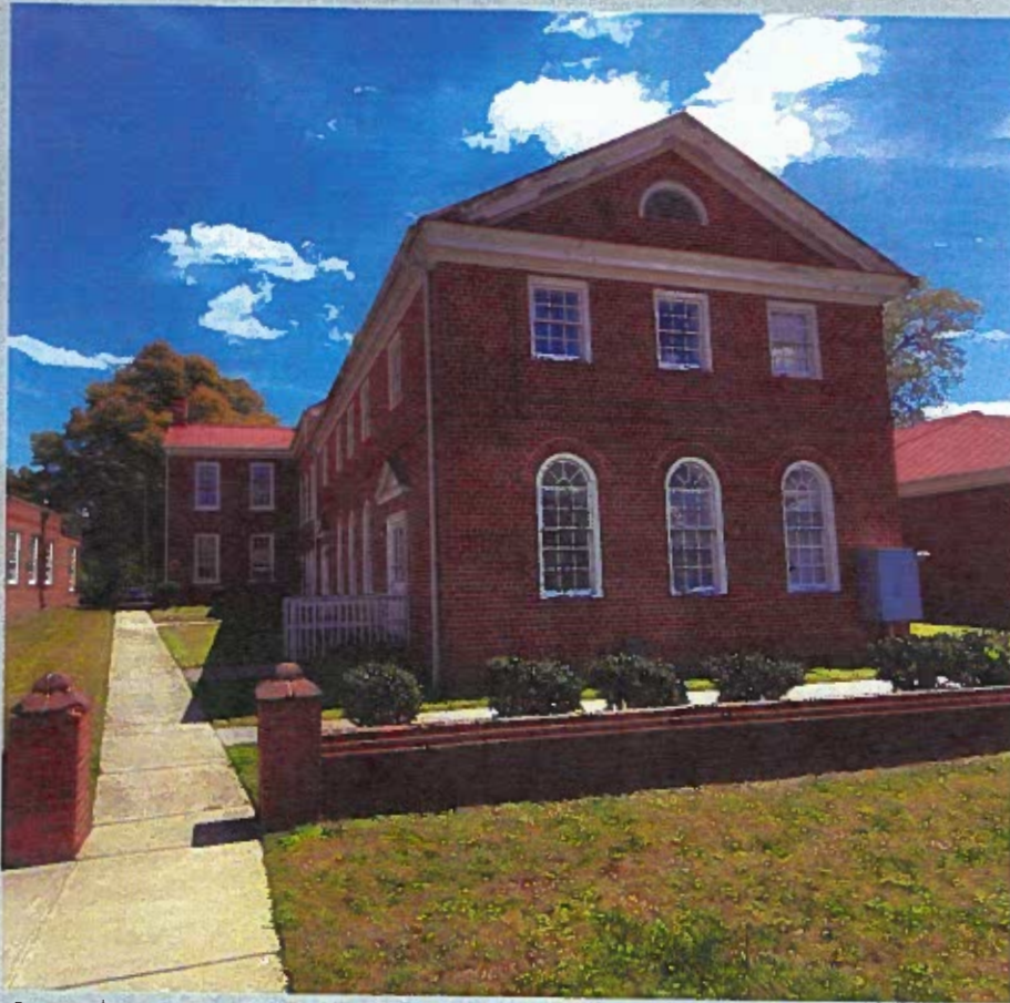
Present-day condition of the 1954 addition from the rear of the courthouse looking North toward the original wings.
