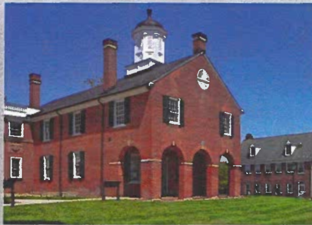
Fairfax County Courthouse, 1799.
