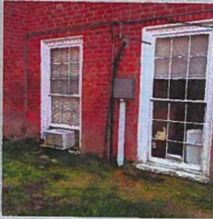
North wall of 1954 addition, showing windows at grade.
