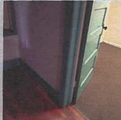
Modern wood over concrete on first floor in the South wing.
