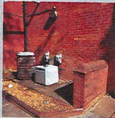
Current conditions within mechanical yard on south wall
