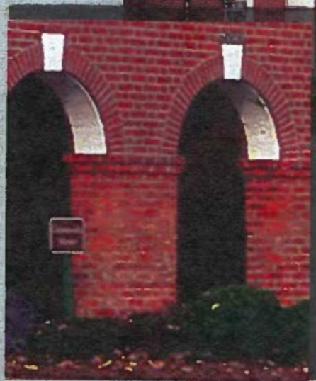
Sussex County Courthouse, 2003, showing repointing and limited damage developing on the lower walls.
