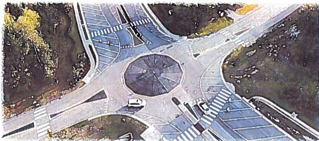
Figure 10- An overhead look at the completed modular roundabout at Otterdale/Hampton Park.
