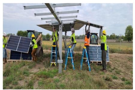
Figure 2 - Crews installing modules on tracker systems
