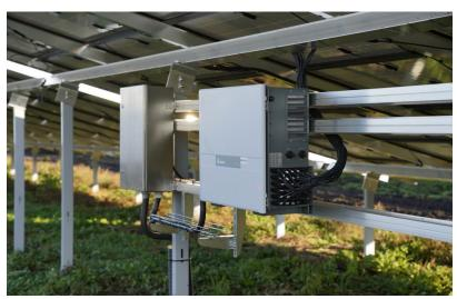
Figure 4 - Example of a string inverter, attached to the tracking array structure.
