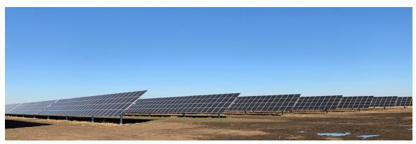
Figure 1 - Solar Arrays mounted on tracker systems
