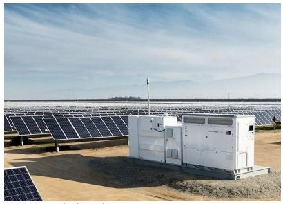
Figure 3 - Example of central inverter
